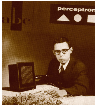
Hardware implementation: Mark I Perceptron
