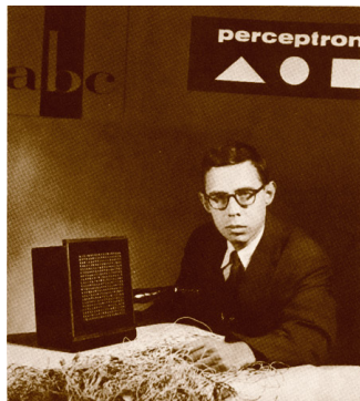
Hardware implementation: Mark I Perceptron
